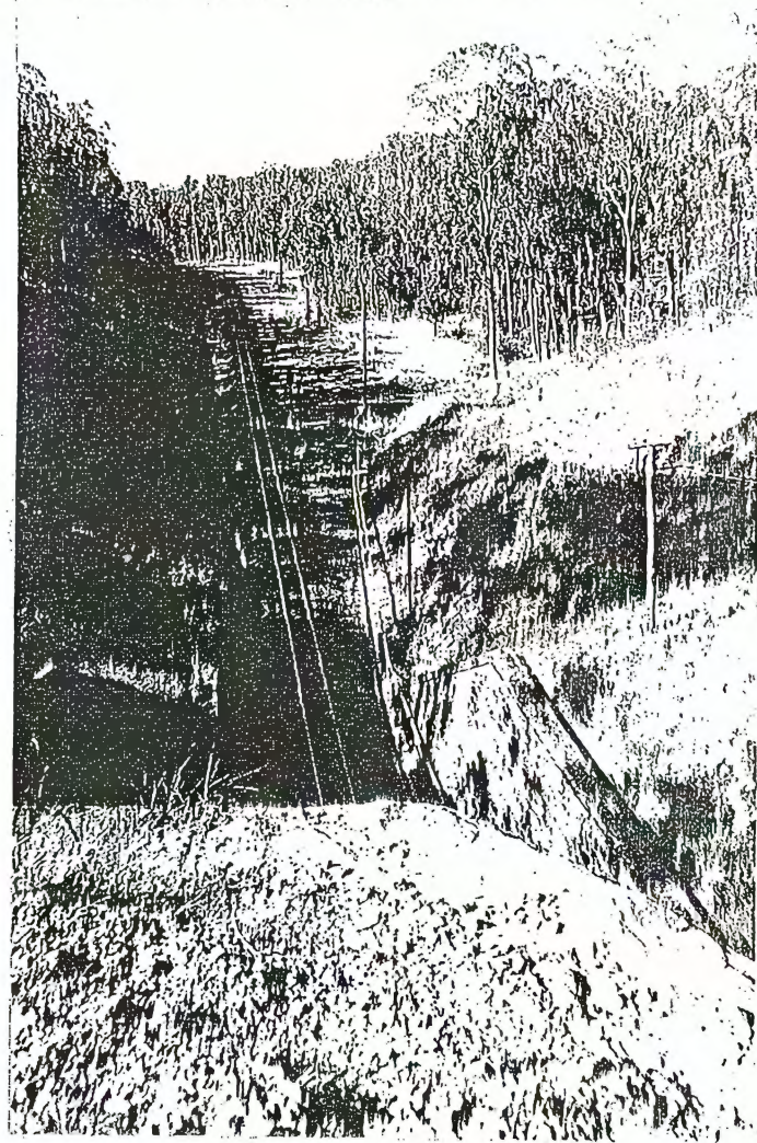
Victoria Tunnel: eastern approach
