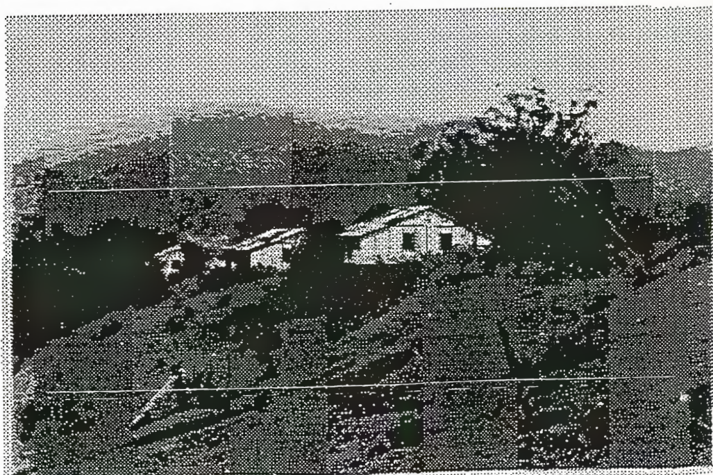
View of three fibro sawmill worker houses (two more obscured)
