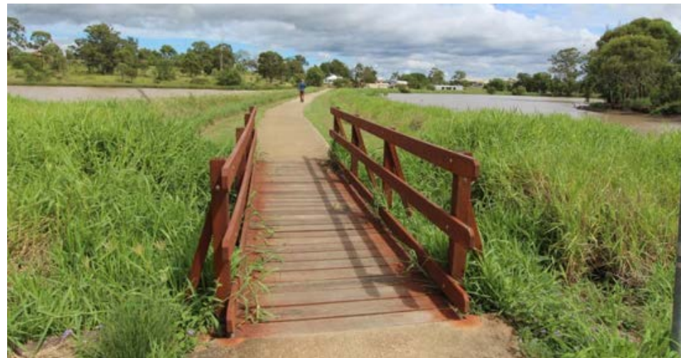
Figure 4-8 Footbridge and the vegetated channel which joins the two lakes
