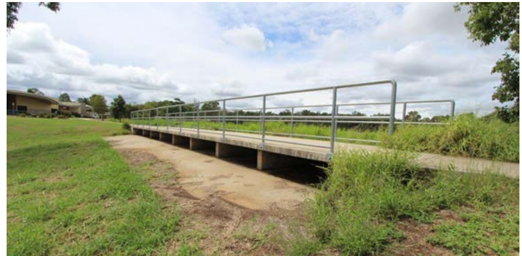
Figure 4-9 Outlet weir and culverts in the north-west corner of Lake Apex
