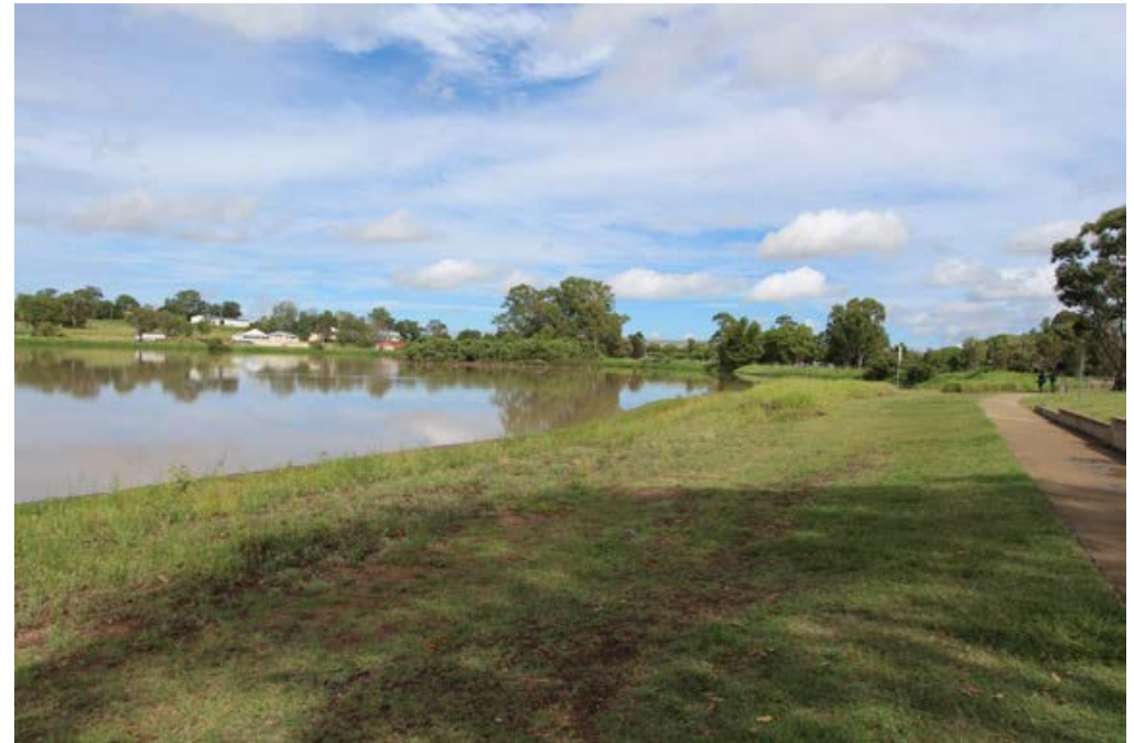
Figure 4-16 Example of poor delineation between riparian habitat and turf around lake edge
