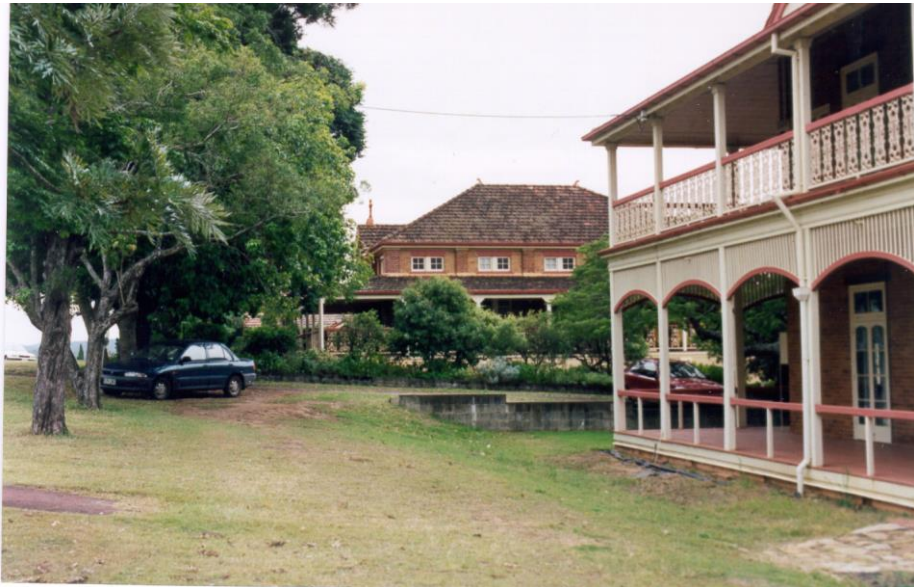
Convent School in background, former convent on right
