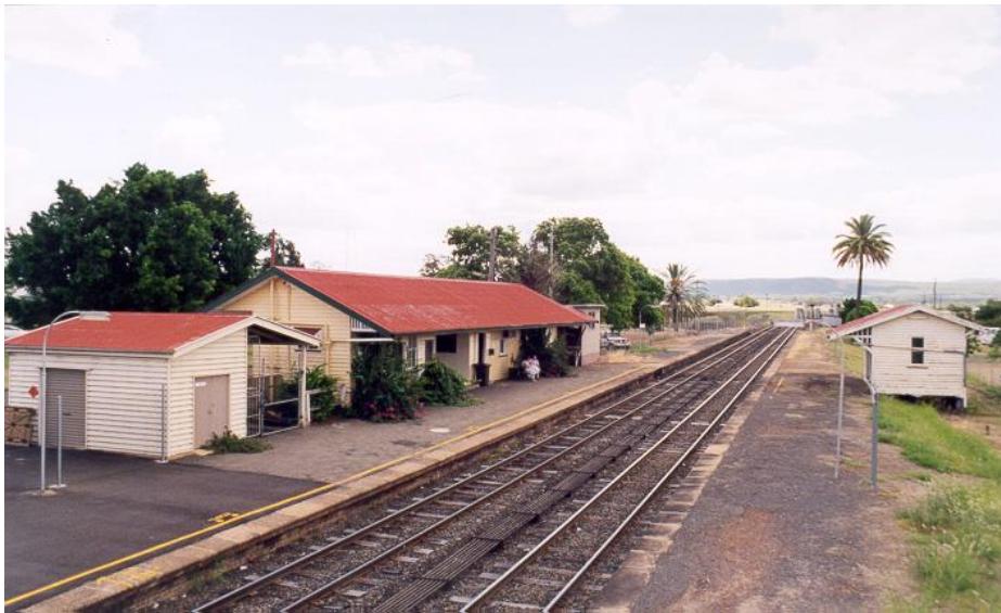
Store, Passenger Station and Waiting Shed
