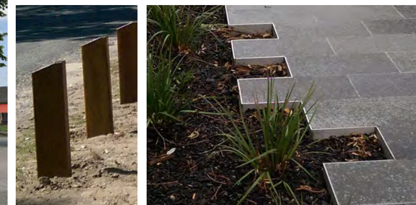
Contemporary street furniture with simple shapes. Preference for hardy materials like hardwood and aluminium/steel to minimise maintenance. Modern edging to accentuate key nodes (business district).
