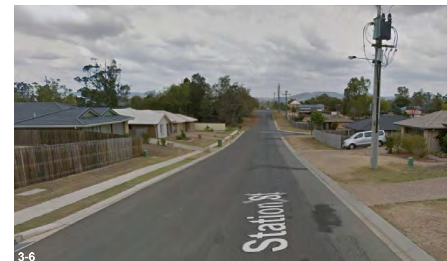
3-6 Existing collector road, Station Street - urban setting at Helidon.
