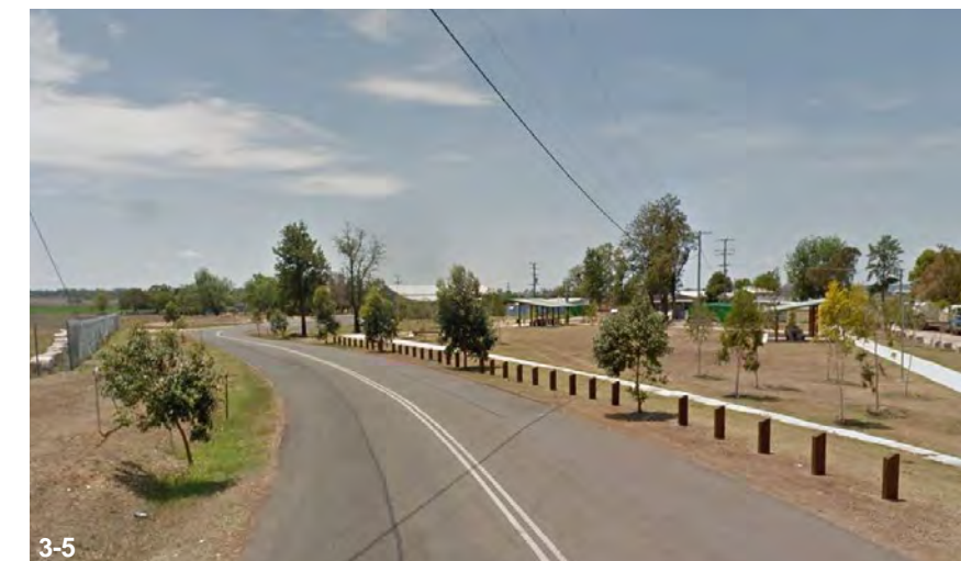
3-5 Existing distributor road, Railway Street - urban setting at Grantham.
