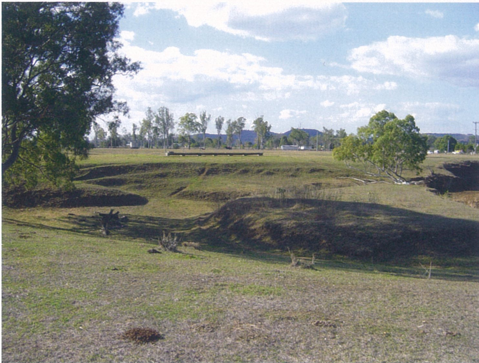
Photo 5. Poor condition of Plain Creek north of the Warrego Highway.
